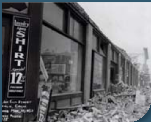
Earthquake damaged storefronts on Broadway and Elm Street.
